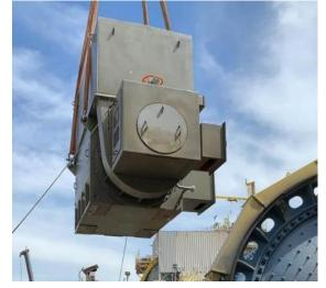
Installation of repaired motor on ball mil - December 2020
