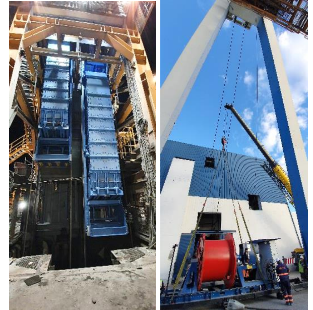
New skips and hoisting rope installed
