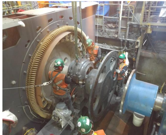
Candelaria Ball Mill 2 motor replacement during Q4/19
