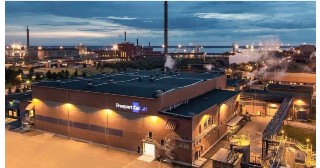
Kokkola Cobalt Refinery
