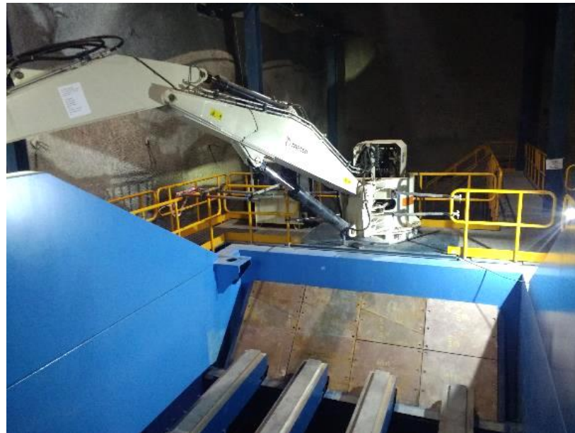
Crusher chamber – rock breaker and hopper
