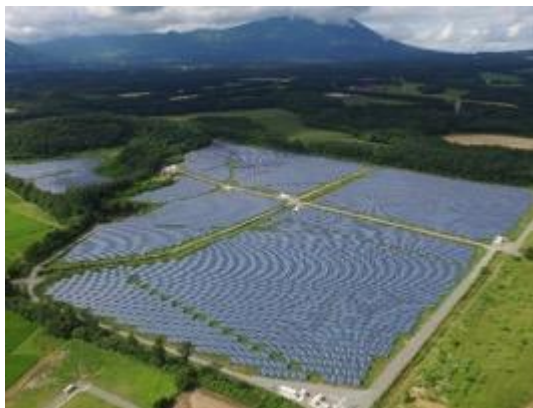
General aerial view of full plant
