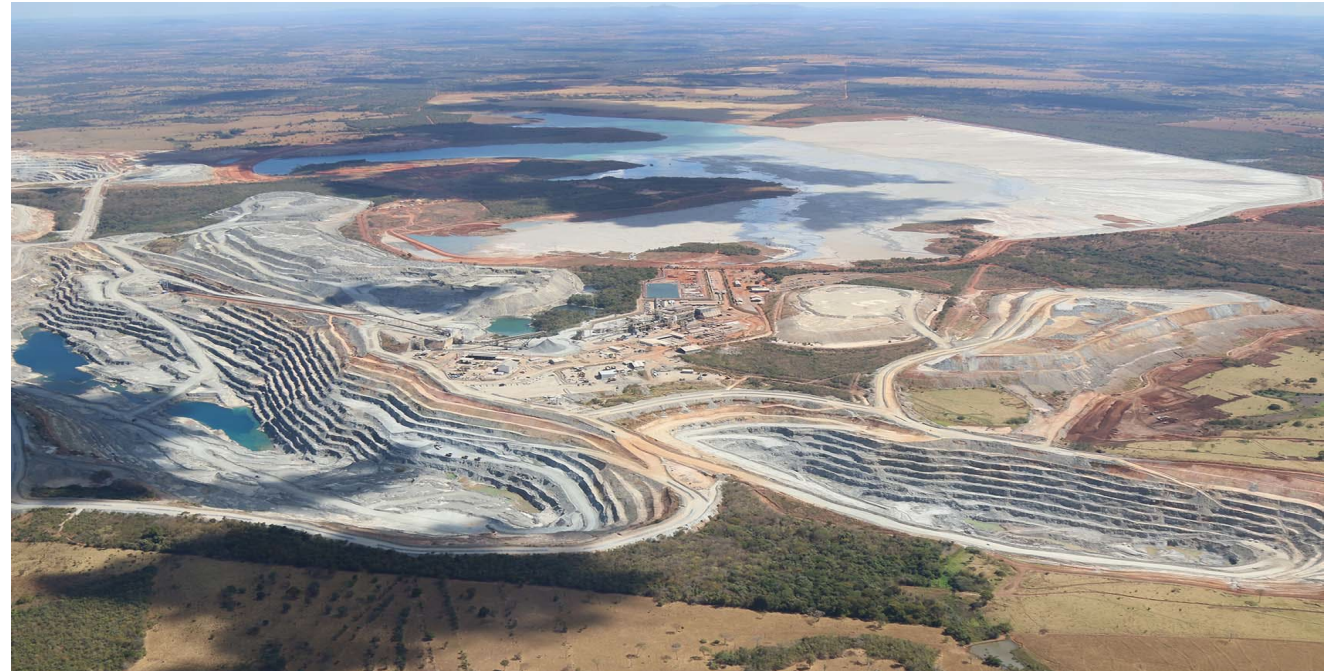
Chapada North and Main open pits in foreground, processing facilities in center, and tailings storage facility in background
