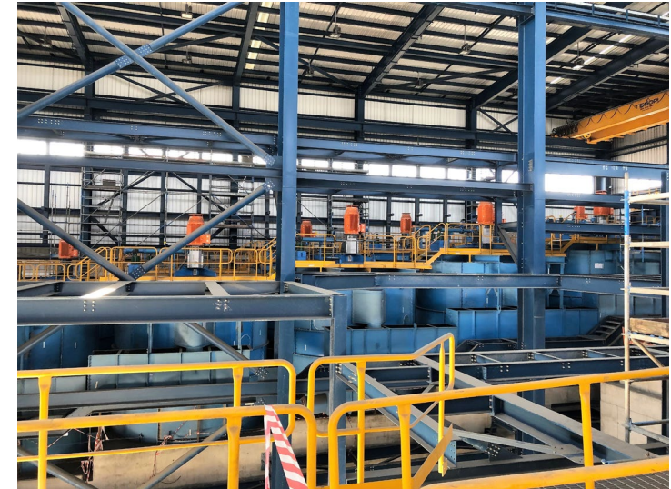
Flotation cells in new zinc plant building
