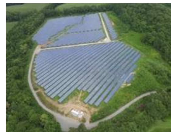
View of the NW section of the plant.
