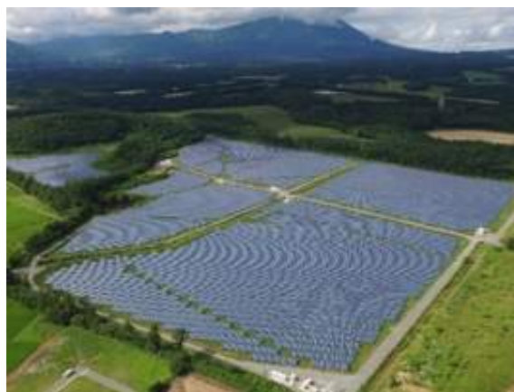
General aerial view of full plant
