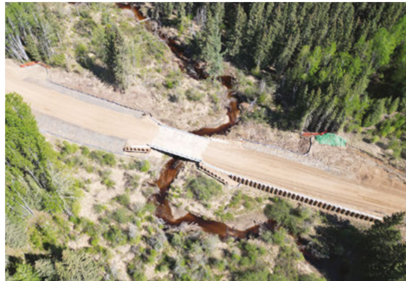
Road access upgrade & bridge enhancement
