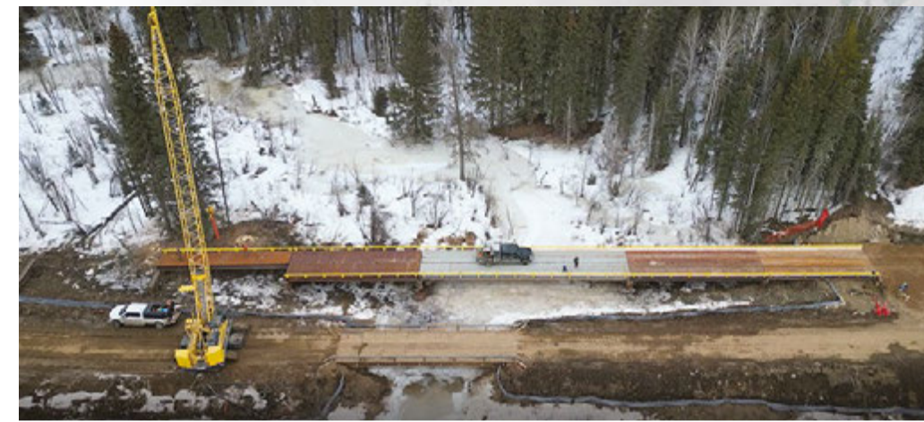
Blackrod - Road Construction
